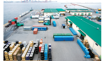
Port-Island Chemicals Center/ Opened in 1998 by borrowing the site from Kobe city. We are working on a large size by scrap & build.
