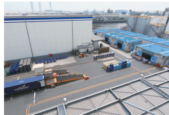
Yokohama Chemicals Center/ The biggest storage houses in Chikko Corporation of East of Japan and also expanded a new warehouse in 2012.
